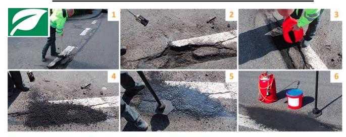
Prepare the area by removing all loose debris and extraneous material from the pothole. The surface to be treated needs to be dry.
