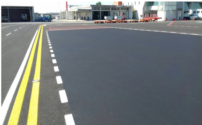
Resin K-EC – treatment of pavement in airport
